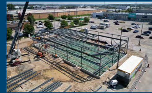
315 Arthur Street South, Elmira ON 13,200 sq. ft.
